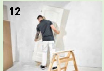
Place the door in an upright position and use wooden blocks or spacers to prevent it from touching the floor and wall if possible.
