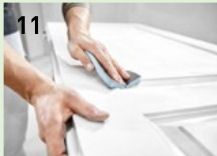
If necessary, resand hard-to-reach areas on profile grooves and transitions again using a hand-sanding block.
