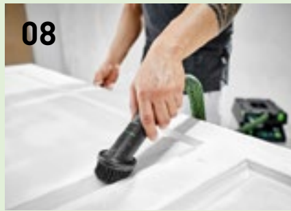
Thoroughly remove dust from the sanded surfaces using an anti-dust and tack cloth for painters or, if necessary, with the mobile dust extractor, a hand tube and suction brush.
